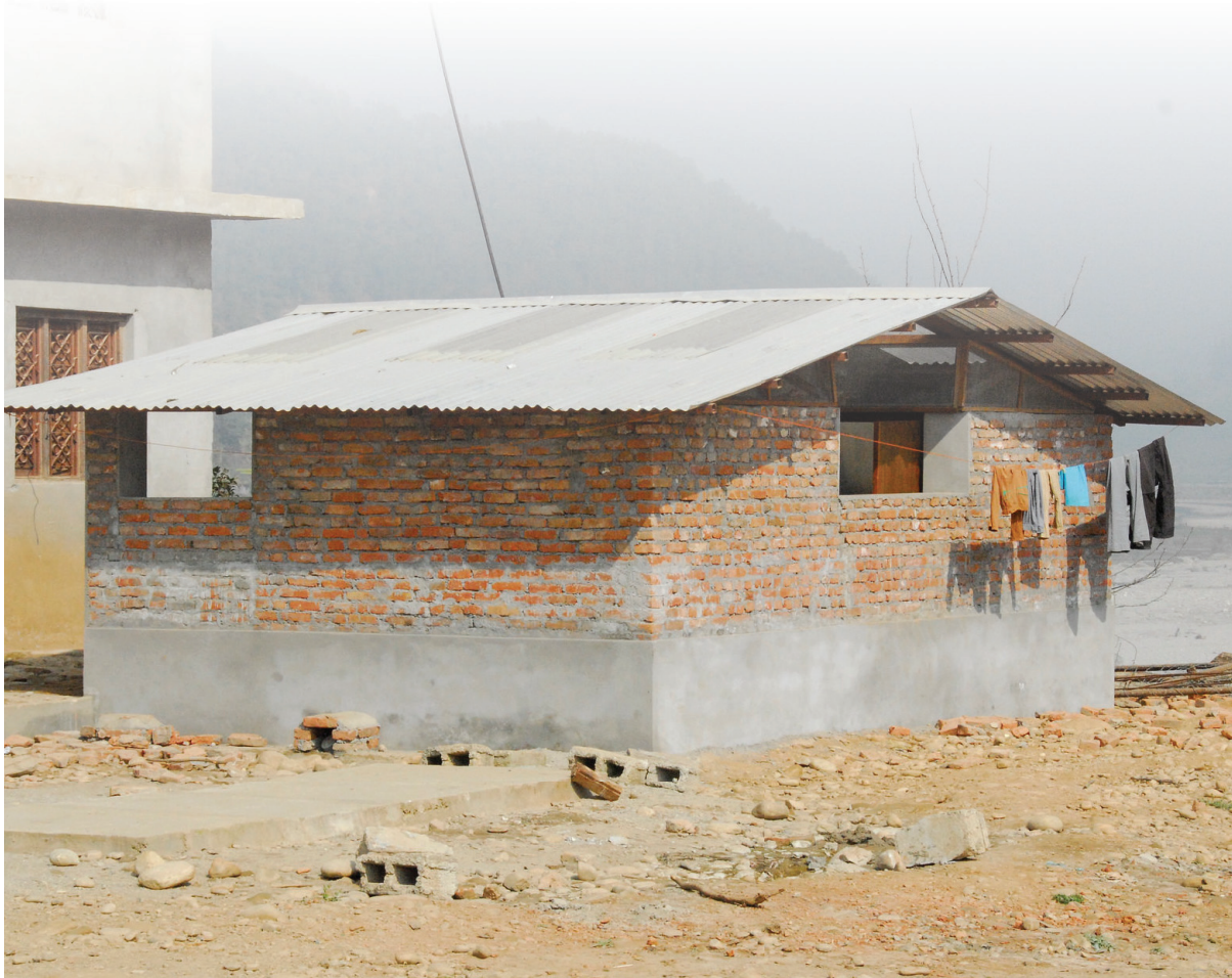
Stage 1 – Completed girls toilet block
