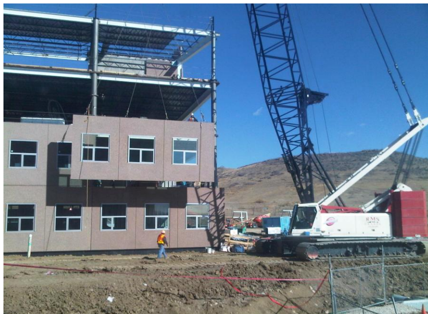
Figure 5–1 Precast wall panels with windows being installed in the RSF expansion
