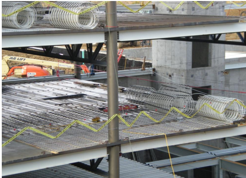
Figure 5–2 Radiant tubing mat installation
