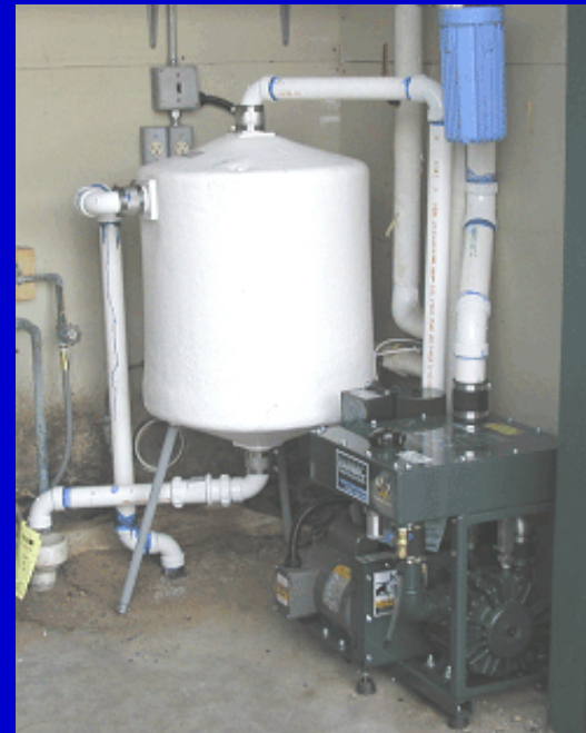
Old Liquid Ring Pump New Dry Vacuum Pump
