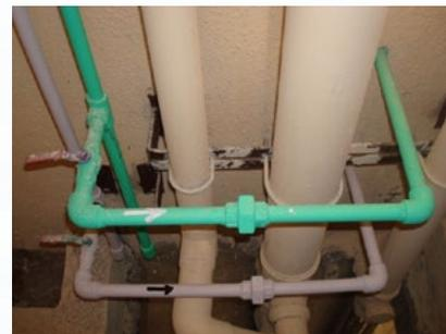
Pipe colour coding and arrow marking.
