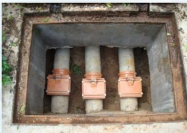
Back water valves on storm drains, before connecting to nalah.
