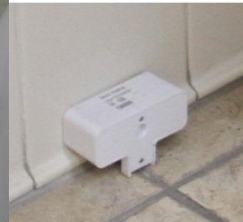
Water Leak Sensor
